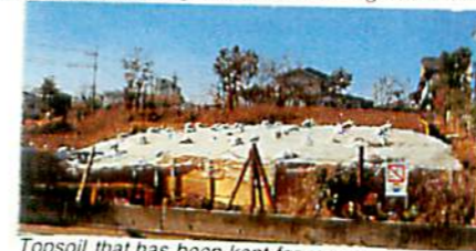
Topsoil that has been kept for re-use
