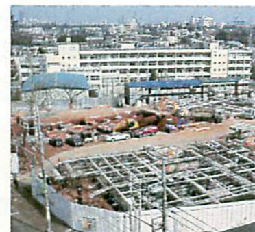
Construction starting at last
