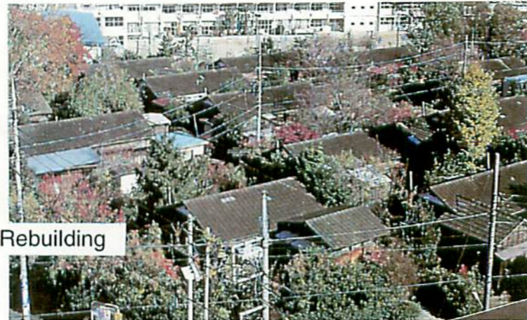
Overview of the houses just before demolition: a site overflowing with greenery
