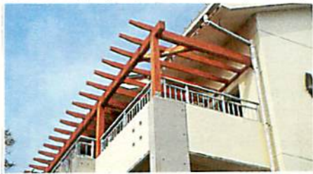
Pergolas shade the uppermost floors
