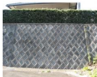
練石積み造擁壁
