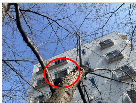
①大枝、樹皮欠損腐朽
