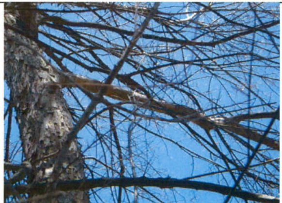
②樹皮腐朽
